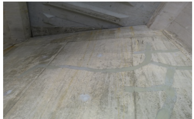
⑪ 균열 0.5mm / 1.5m (보수완료)
