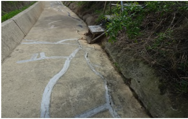
⑪ 침하균열 cw=4.0\text{mm} / 4.0\text{m}
