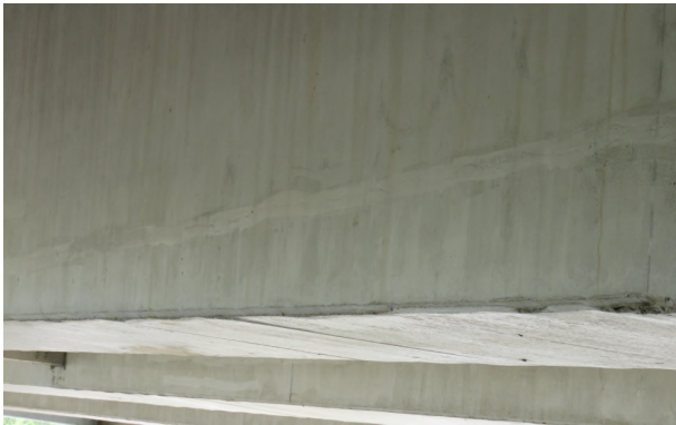
② 균열 (0.3mm미만) cw=0.2mm / 4.3m (보수완료)
