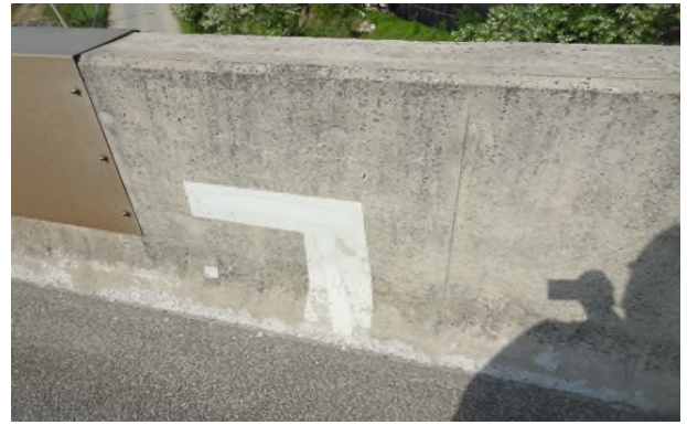
② 균열 (0.3mm미만) cw=0.1mm / 0.4m (보수완료)
