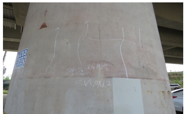
⑭ 망상균열 ( 0.3\text{mm} 미만) cw=0.1\text{mm} / 1.0\text{m} \times 1.2\text{m}
