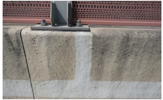
② 균열 (0.3mm미만) cw=0.1mm / 0.5m (보수완료)
